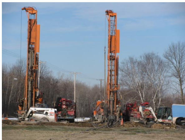
Geothermal well drilling for the Franchere Education Center
