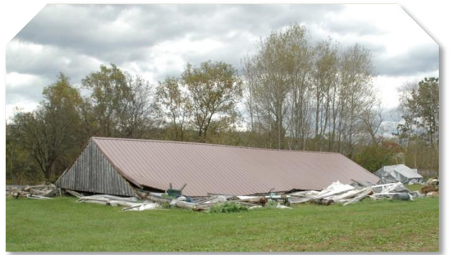
Collapsed pole barn at Mabee Farm after Hurricane Irene.
